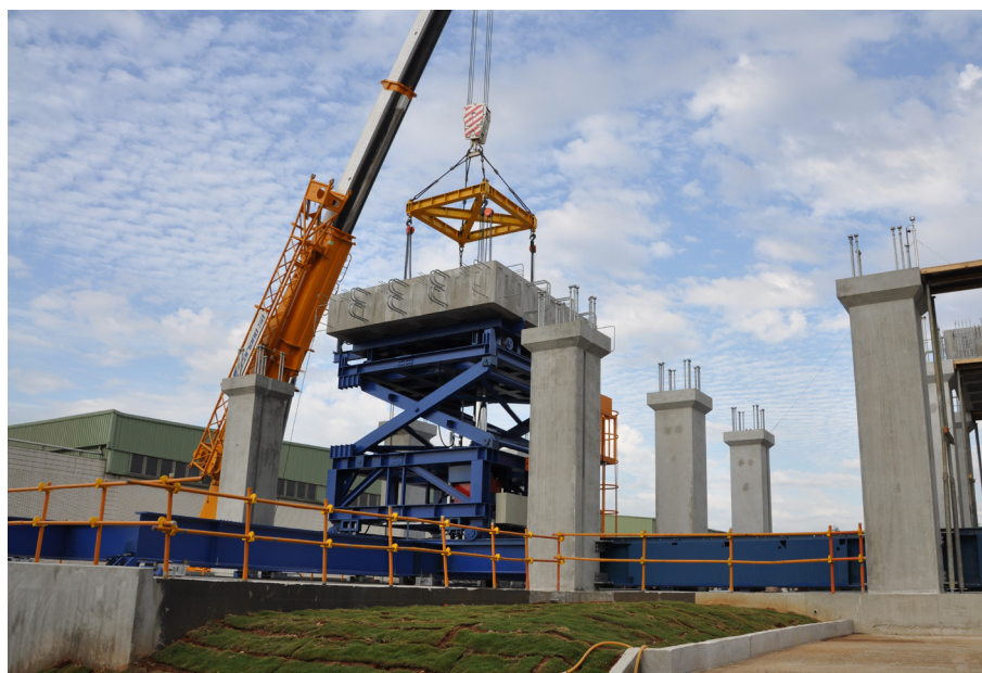
▲ Inventive feature -Mobile installation equipment for waffle slabs
